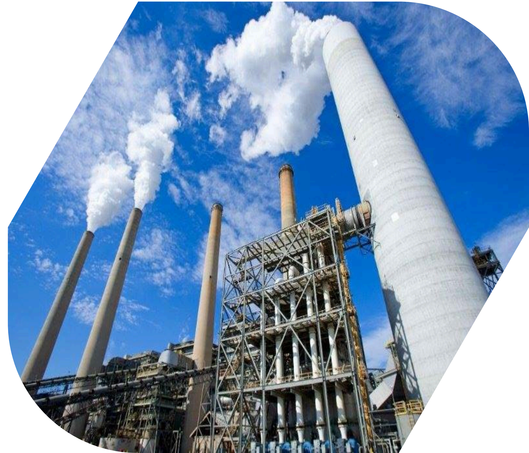
Winyah Generating Station (Photo from Santee Cooper)
