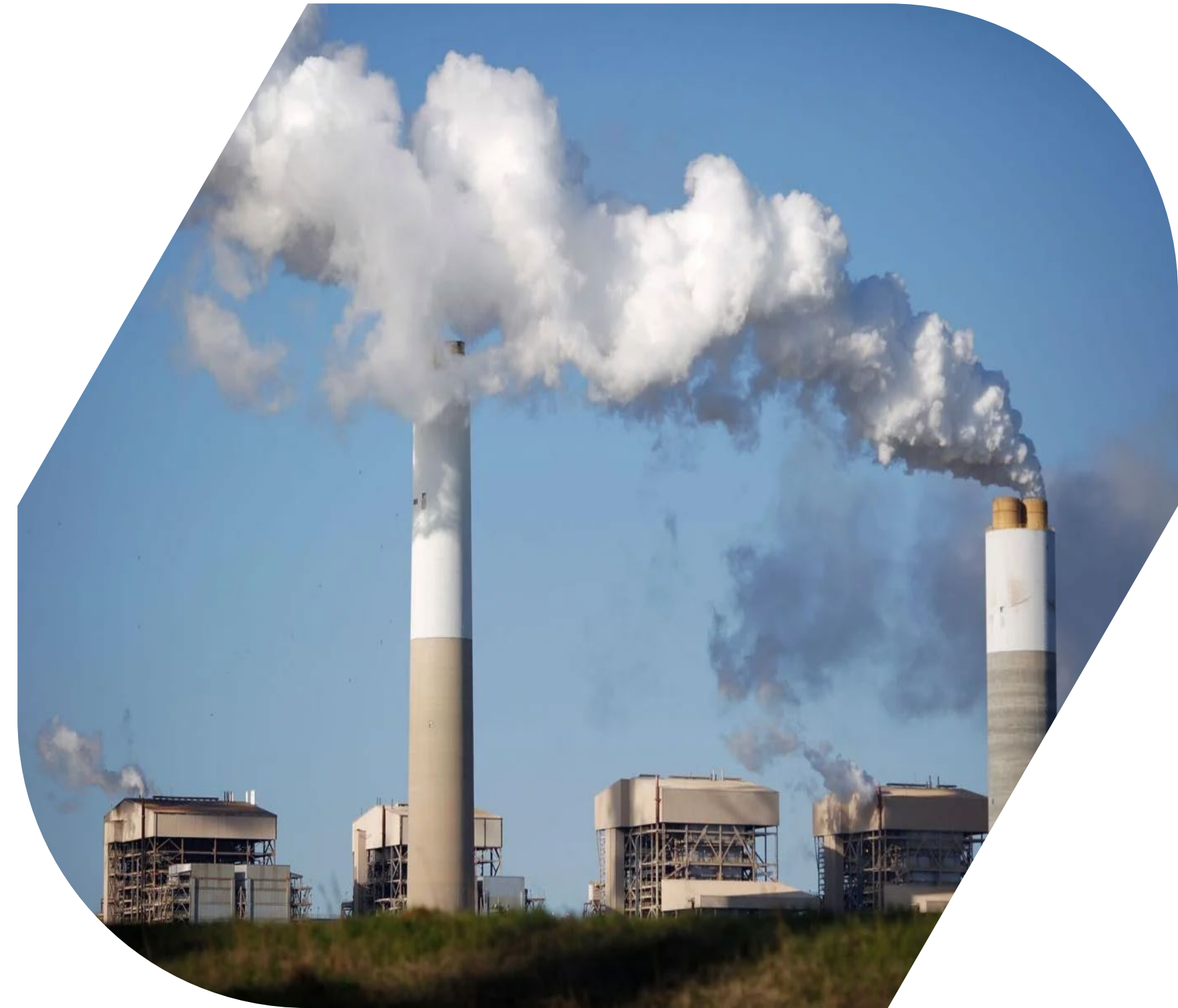
Cross Generating Station (Photo from Santee Cooper)
